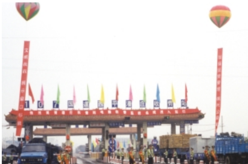
Cheung Kong Infrastructure is involved in the construction of National Highway 107 in Henan Province, China. (Our holding valued at £1.1m.)
