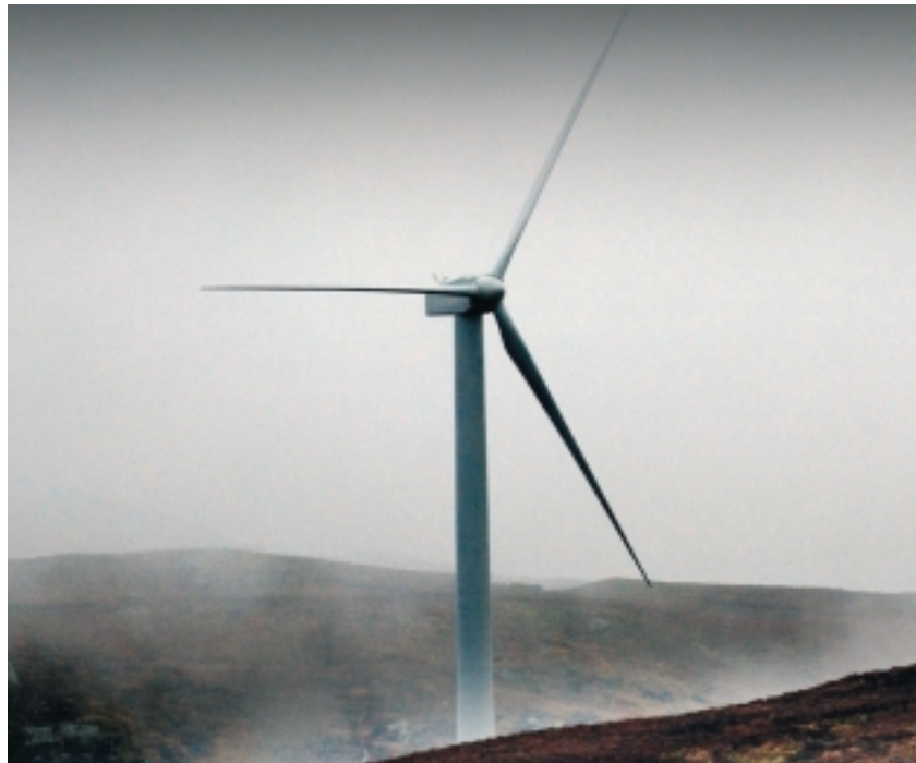
ScottishPower leads the way in alternative energy resources such as wind generation. (Our holding valued at £7.7m).
